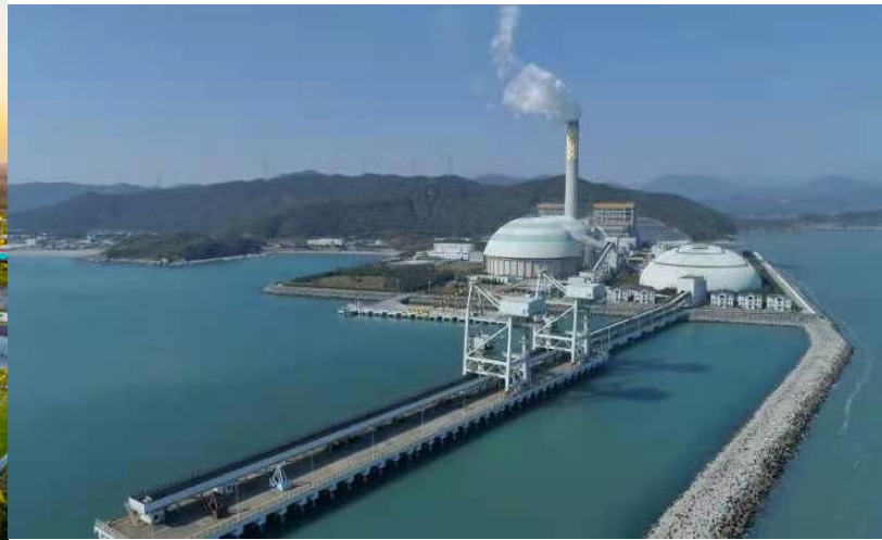
Haifeng Thermal power plant in Shenzhen
