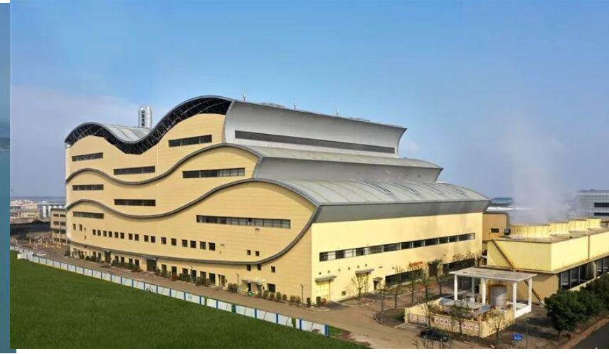
Xiaoshan district sludge TP in Hangzhou
